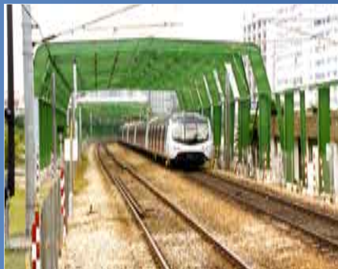
Partial enclosure designed with assistance of NoiseMap
